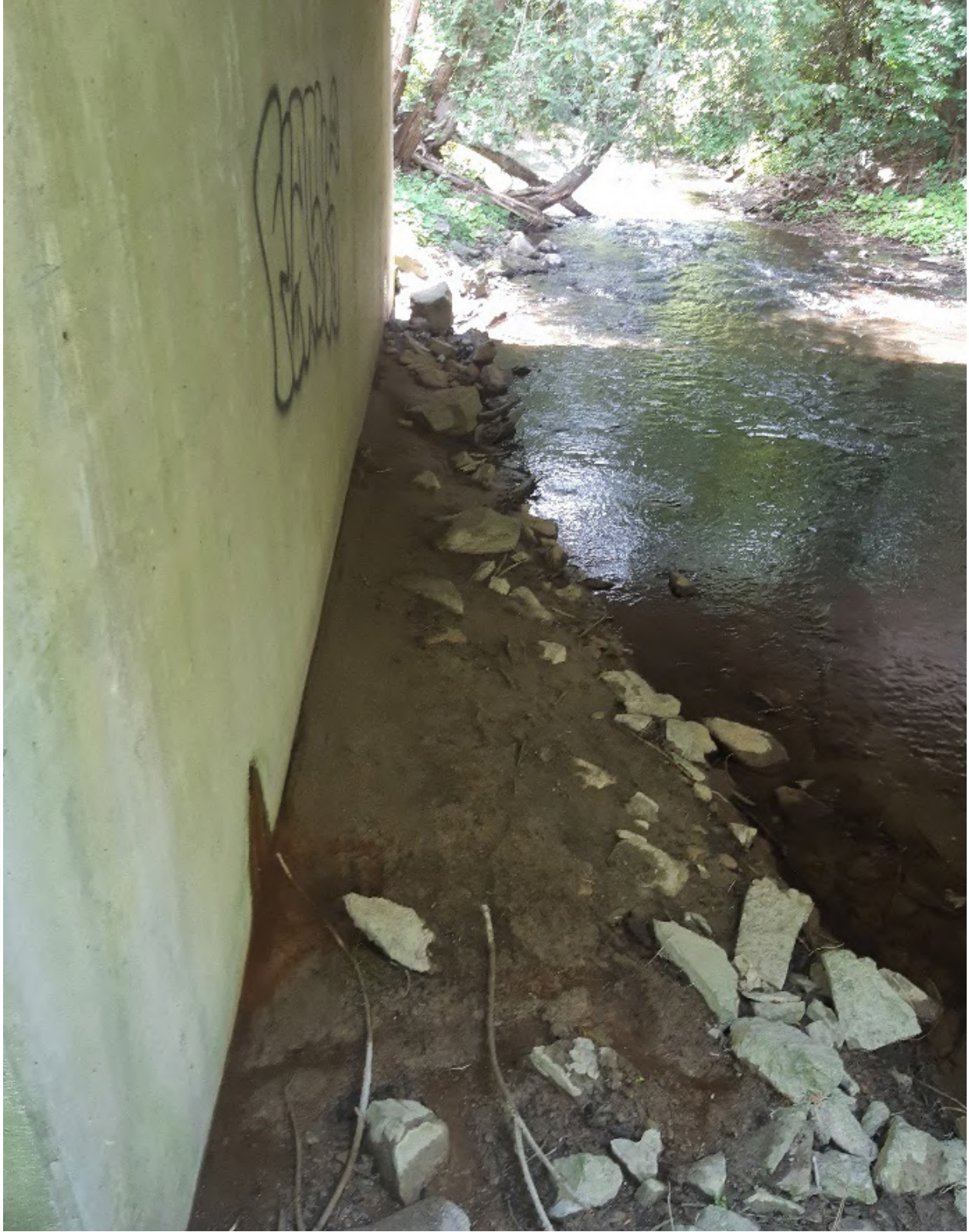
Site 6: Westney and Concession road 8; mud berm along riparian pathway for wildlife passage. A wider pathway would be preferred.
